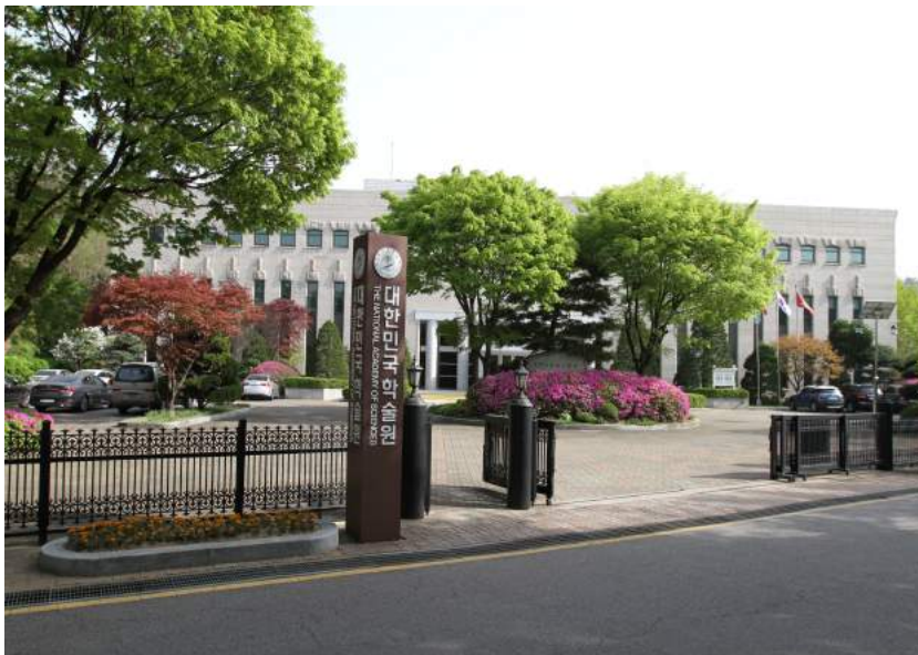
The NAS Building
